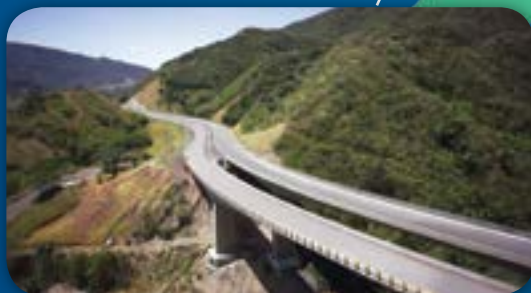
Ruta del Sol (Sun Road) Toxement and Euclid Chemical
