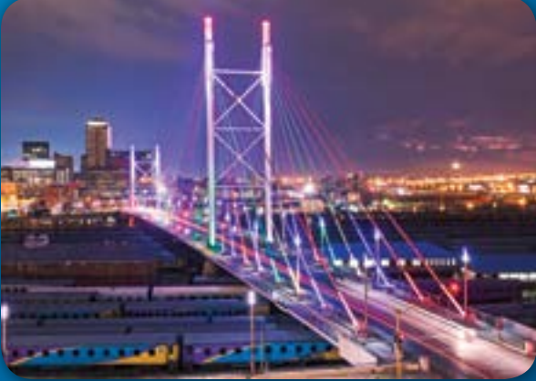
Nelson Mandela Bridge Tremco and Carboline
