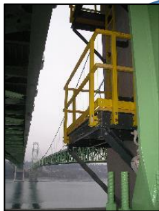
Tacoma Narrows Bridge Protective FRP Washington, USA
